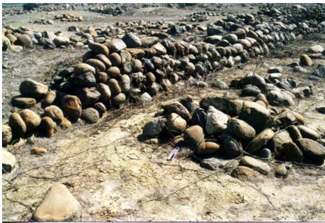
Fig. 5 Looking downstream at the Muralla Pircada, stockpile of cobbles and boulders in the foreground used for construction or repair, scale is 20 cm
