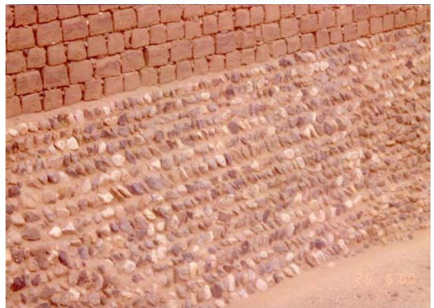
Fig. 7 Well-rounded, well-sorted, imbricated cobbles used to line the bottom of the reservoir at the Chimú site of Chan Chan, Moche Valley, northern Perú
